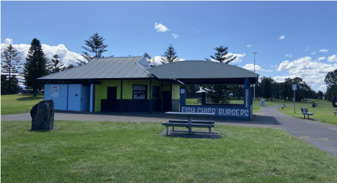
Figure 12 - Existing kiosk due for upgrade
