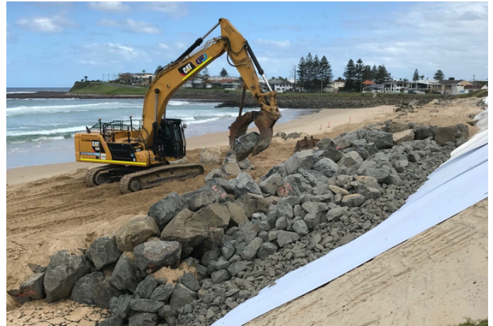
Reconstruction of a new seawall/revetment wall at Warilla Beach.
