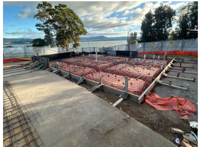
Mid-construction of a new amenities building at Boonerah Point, Mount Warrigal.
