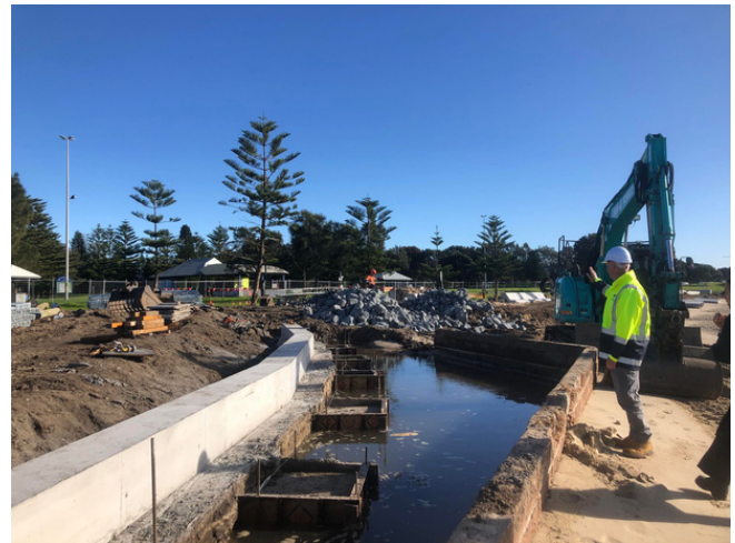
Mid-construction, Stage 2 of the promenade renewal at Reddall Reserve, Lake Illawarra.
