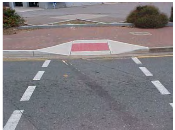
▲ Example of a compliant kerb ramp
