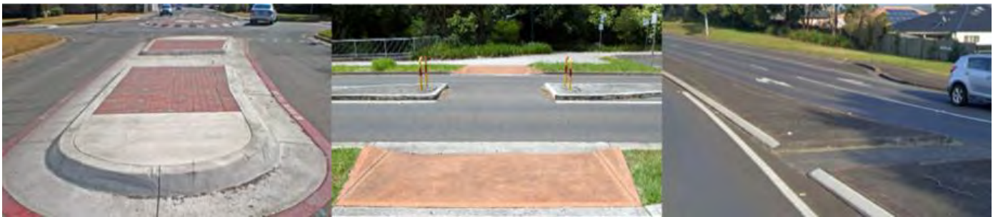
▲ Median, pedestrian refuge and splitter island
