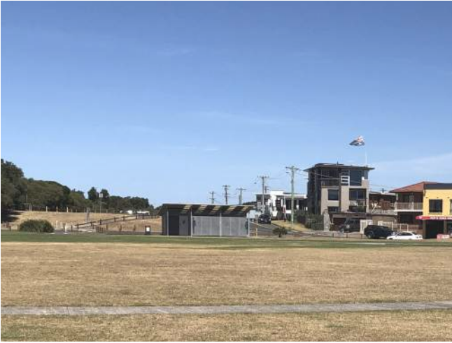
13. Accessible Toilet Block – Constructed (2013)
