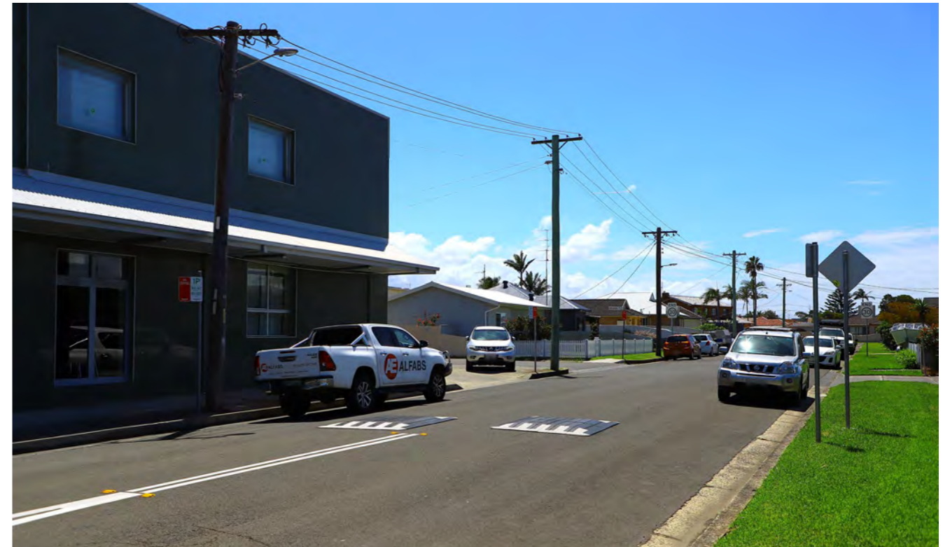
Figure 6.33: Speed cushions on Susan Avenue in Warilla
