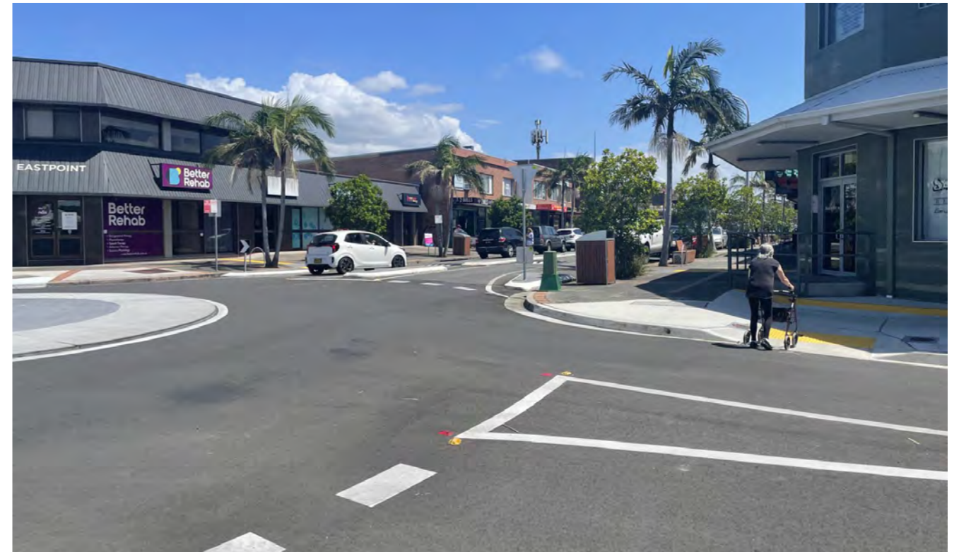
Figure 6.31: Upgraded kerb ramps on George Street in Warilla
