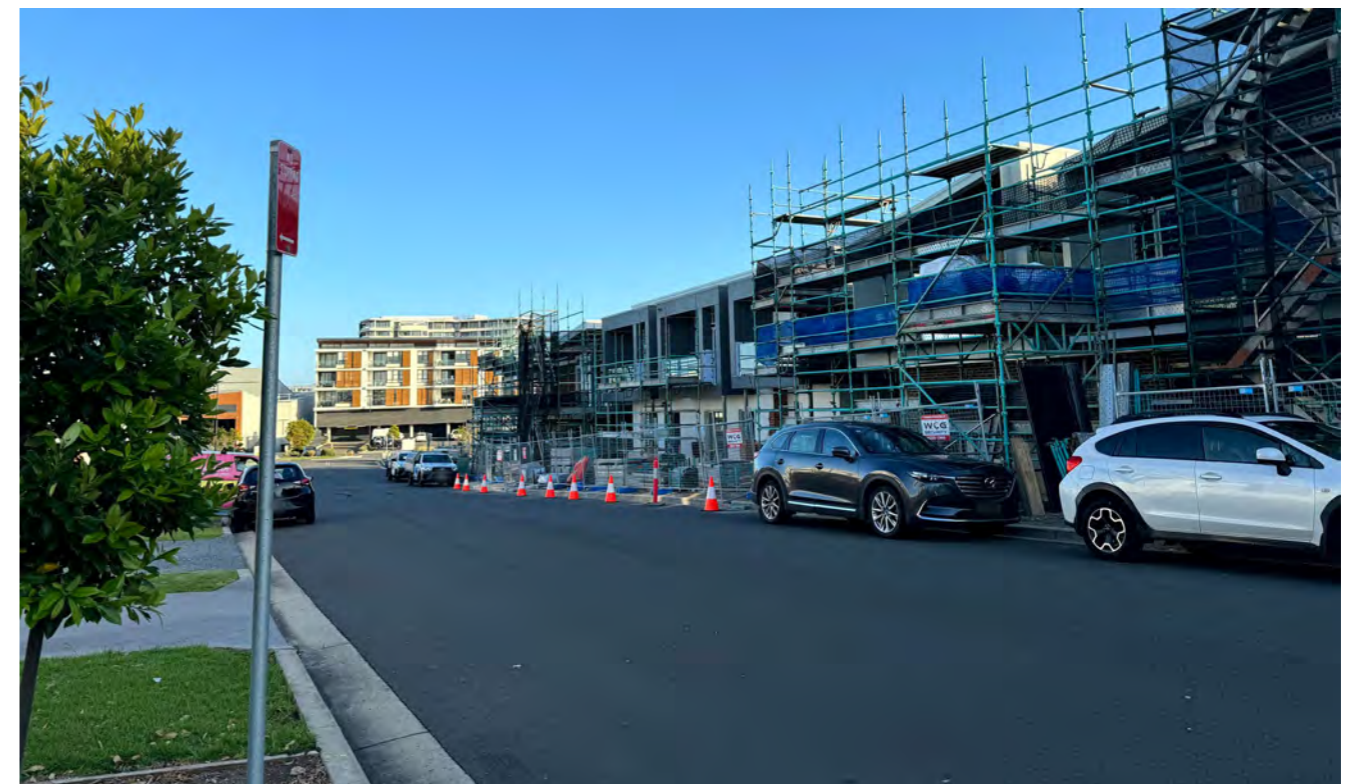
Figure 6.13: Construction projects and temporary traffic management in Shell Cove
