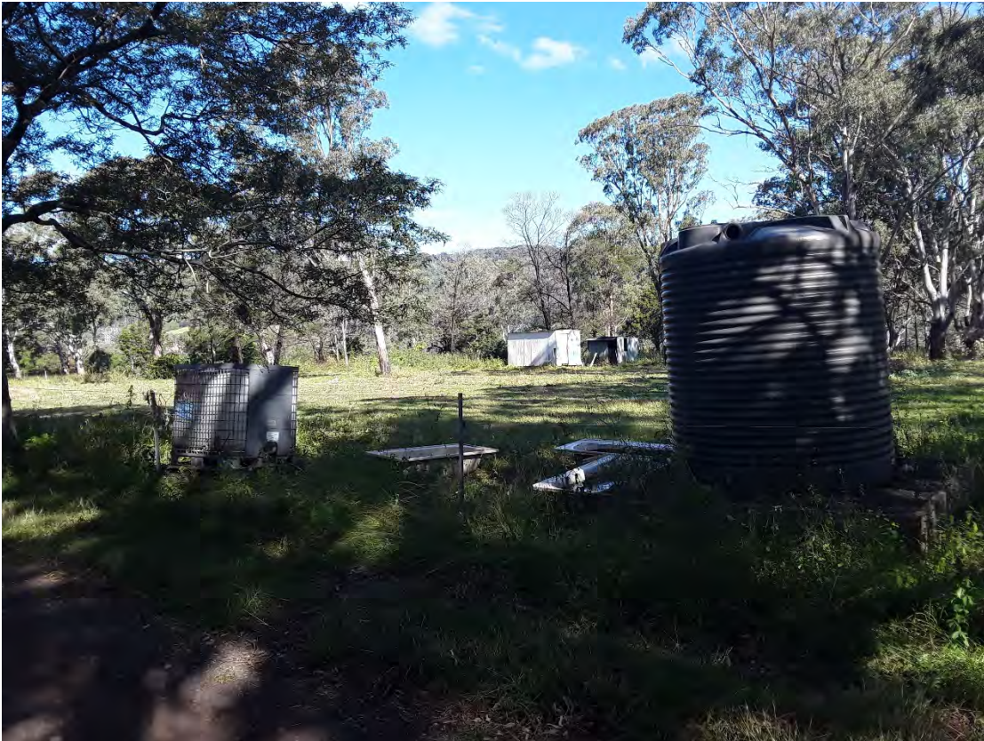
Photograph 1 – Tanks and structures in northern site areas
