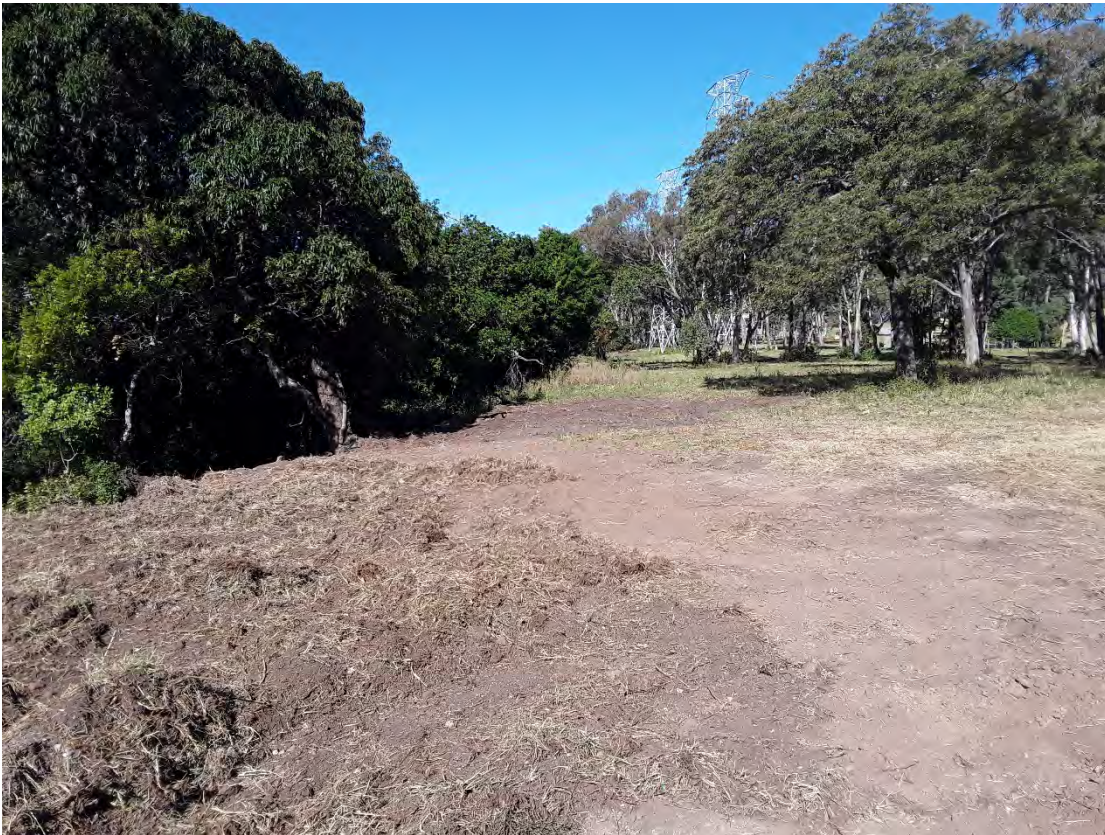
Photograph 8 – Recently emplaced fill, foreground, looking south along eastern edge of ridgeline
