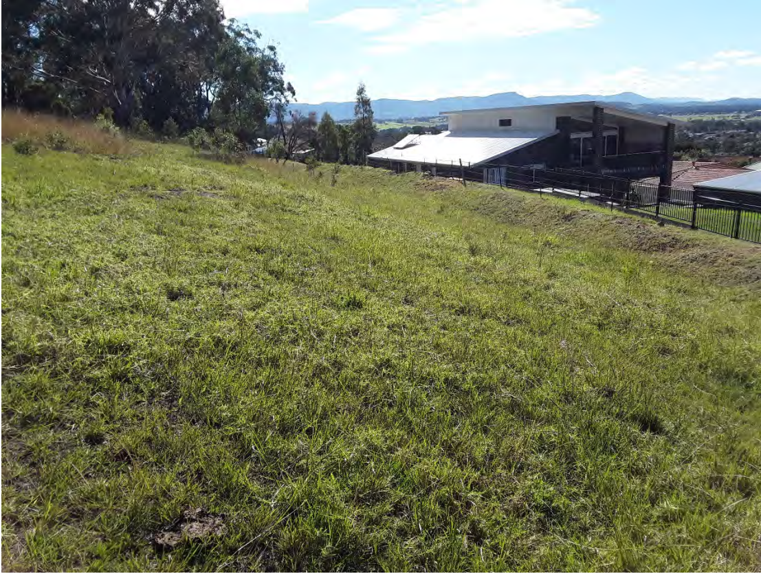
Photograph 2 – Swale constructed on eastern boundary.
