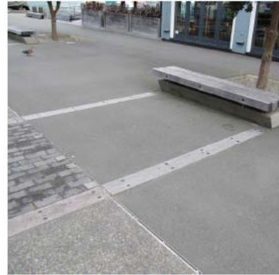
BANDING INLAID TO PAVEMENT
