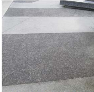
FLOAT FINISH AND SHOTBLAST FINISHES
