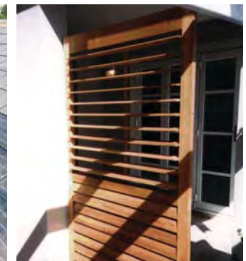
Operable timber louvres for sunshading and privacy
