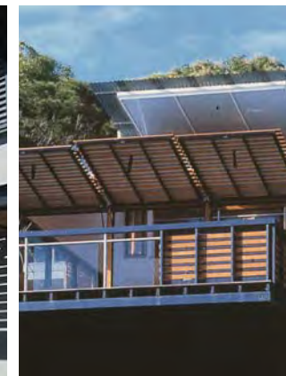
Operable shutters for cross ventilation
