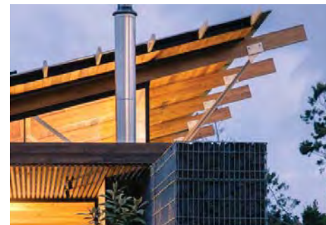
Low pitched skillion roof form
