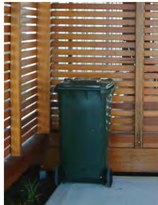
Screened refuse storage
