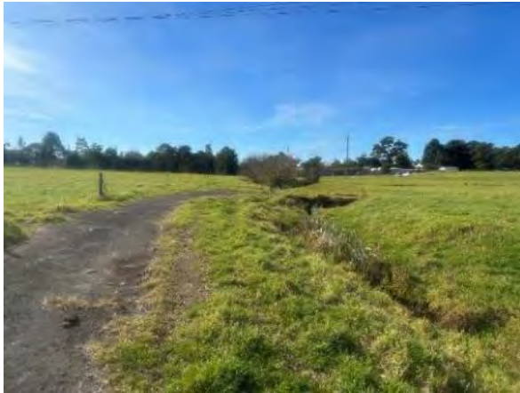
Figure 67. TWE_PAD2 asphalt vehicle access track and crossing of Hazelton Creek looking east.
