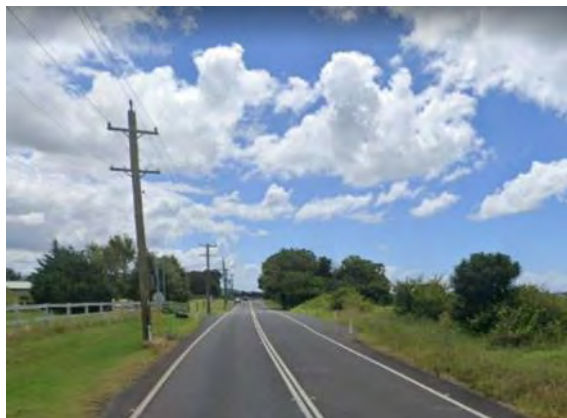
Figure 71. View along Illawarra Highway facing northeast
