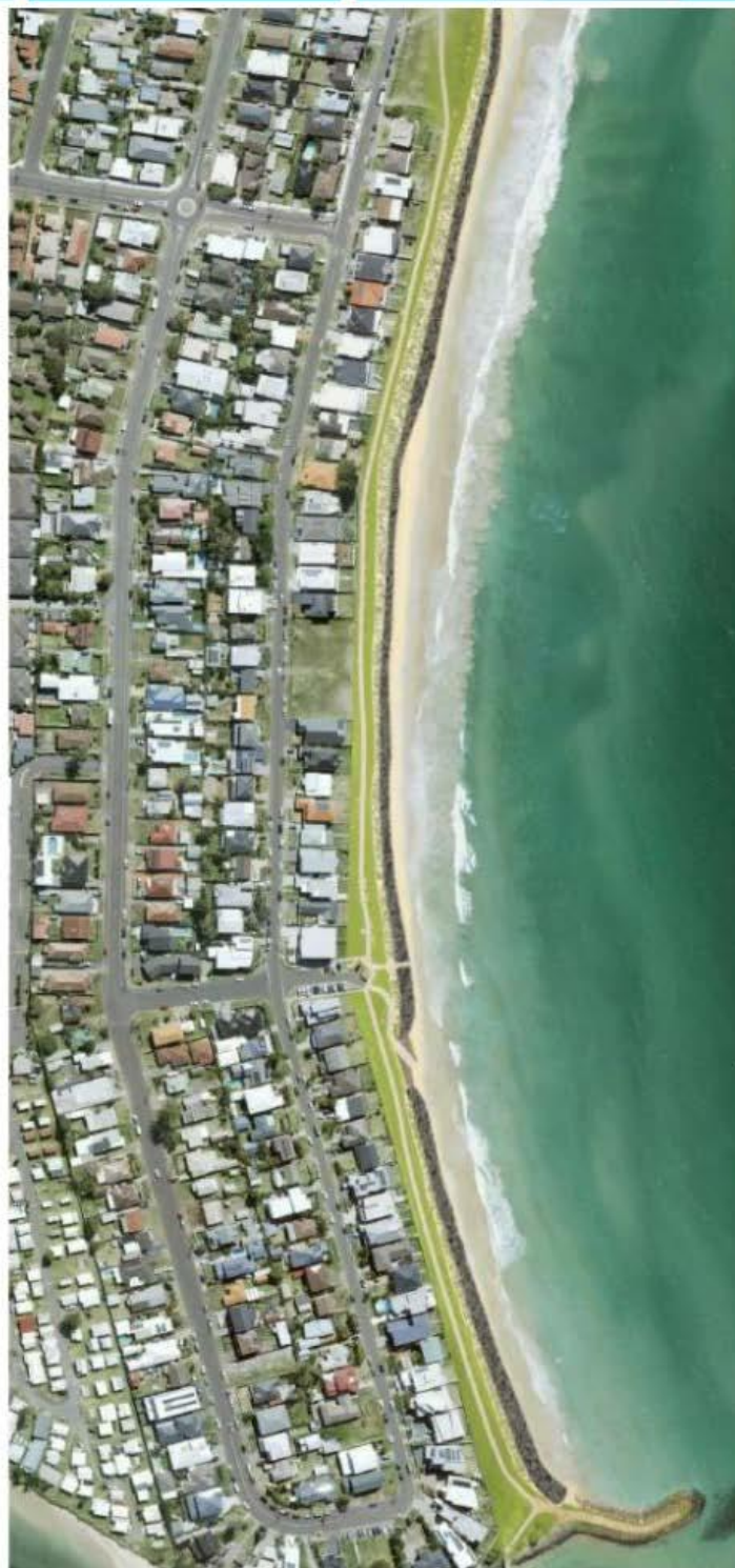
Figure 1 – Aerial Image of the new seawall
