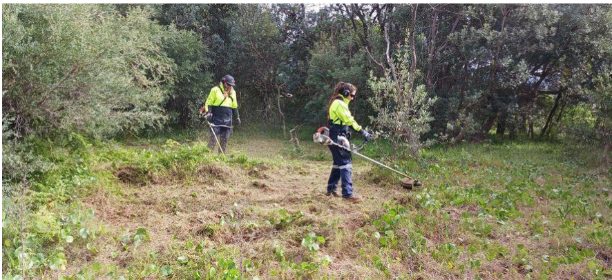
Figure 5 Site preparation, slashing weeds
