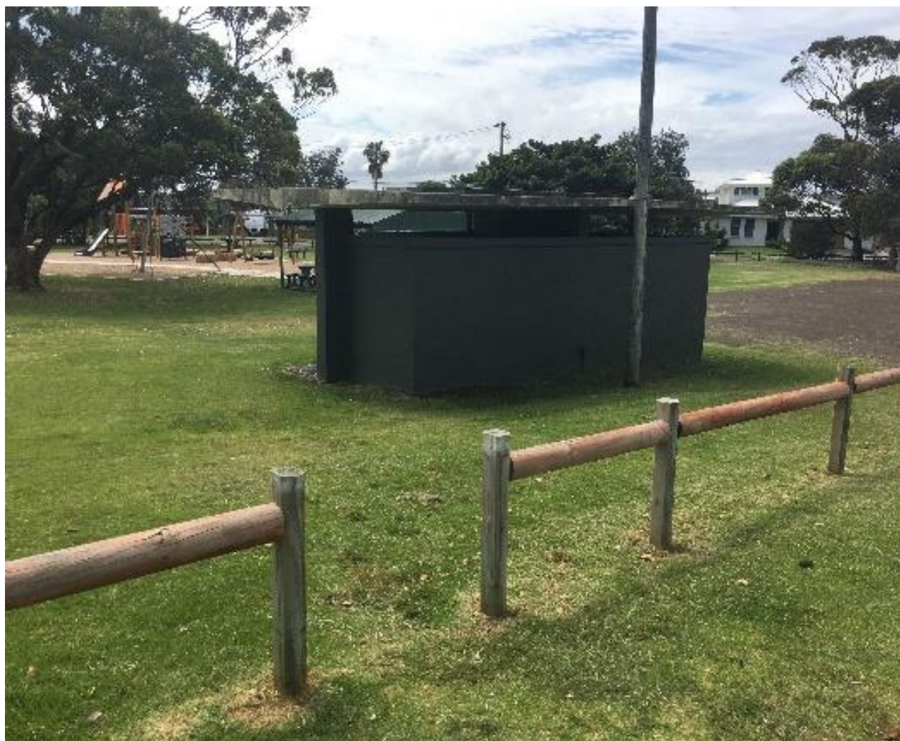
Picture 2: No accessible paths of travel to infrastructure
