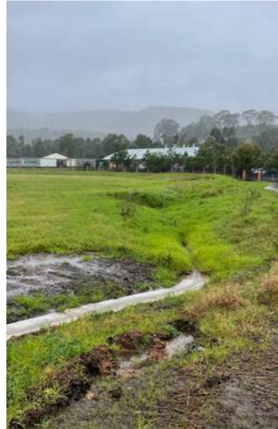
Drainage swale on site
