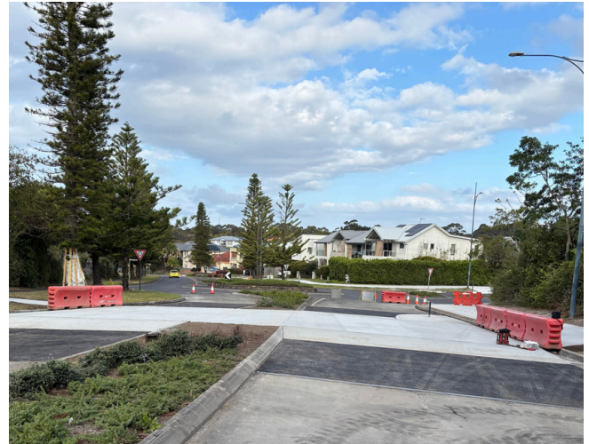
Safety upgrades on Cove & Harbour Boulevard, Shell Cove currently underway.
