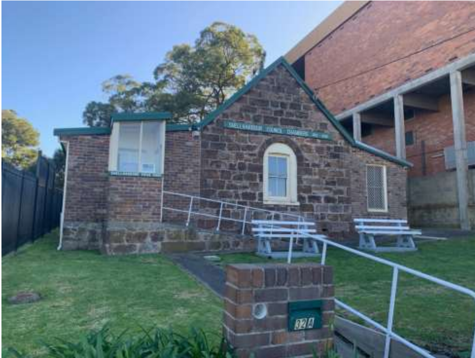
Figure 5 - First Council Chambers, Shellharbour.
