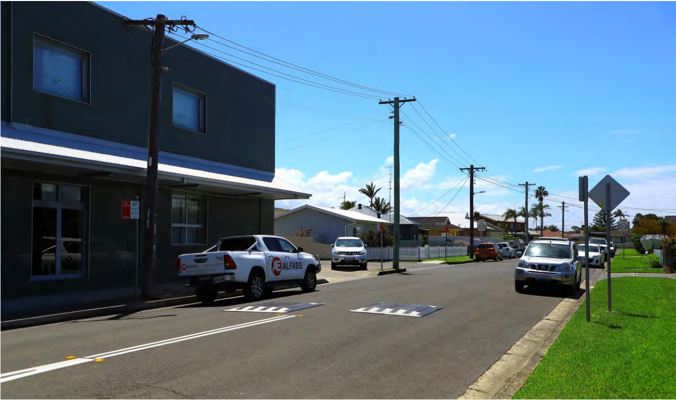
Figure 6.33: Speed cushions on Susan Avenue in Warilla
