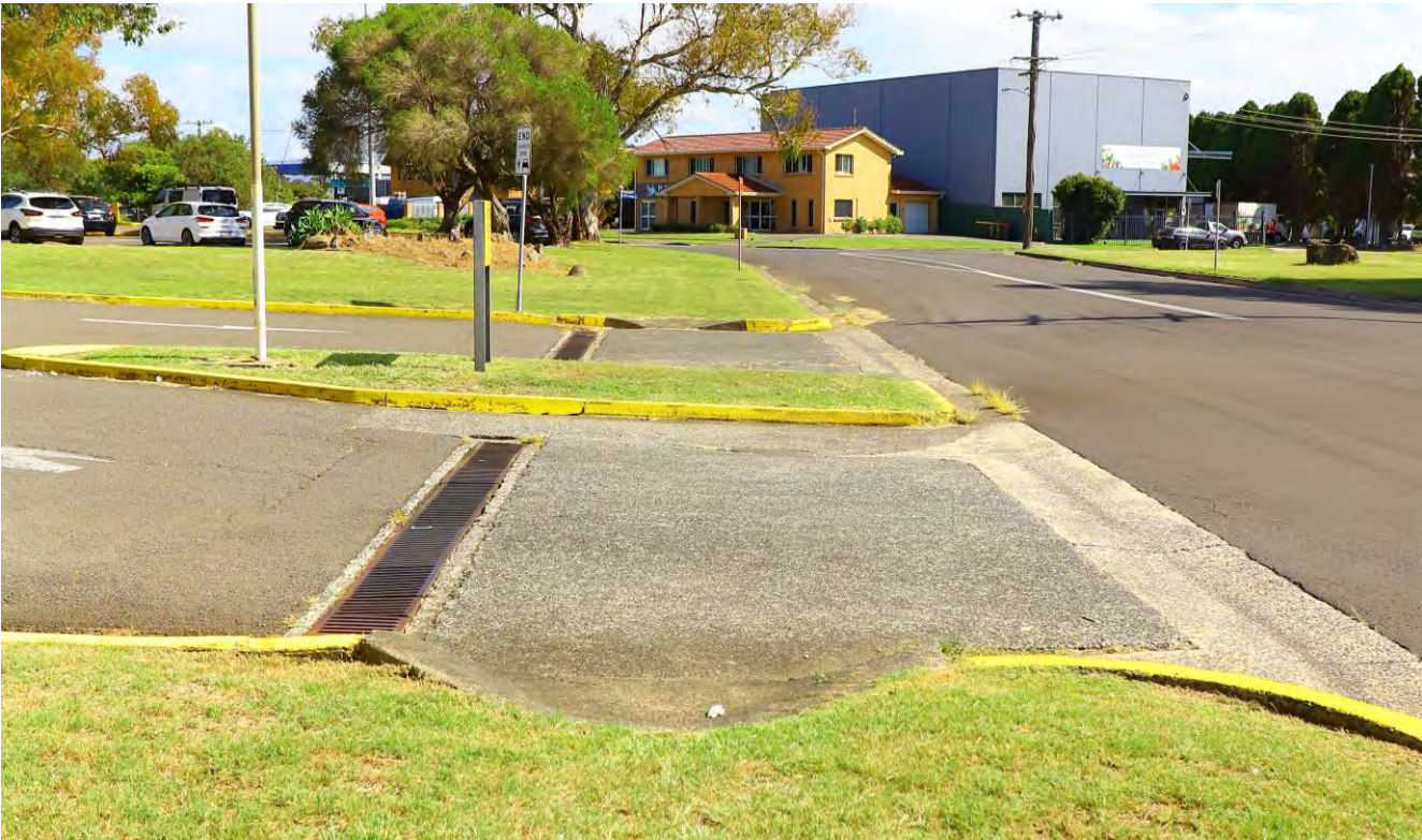
Figure 6.39: Missing footpaths and pram ramps across the car park access to the Warilla Grove Shopping Centre
