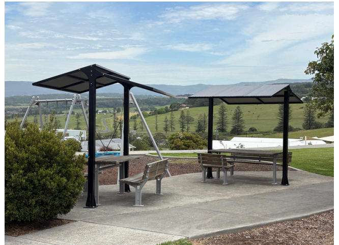
Two new shade shelters have recently been completed at Andromeda Reserve, Dunmore.
