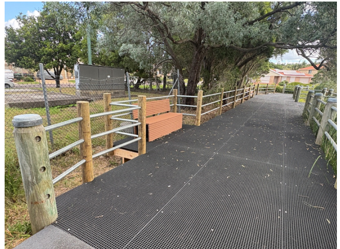
The pedestrian bridge renewals at Grainger Reserve in Flinders and Brindabella Wetlands at Shell Cove are now complete.
