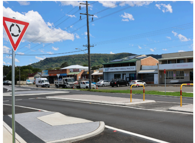
Road and pedestrian safety improvements at Terry Street, Albion Park, are now complete.
