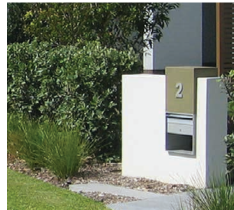
Pier and landscape front fencing
