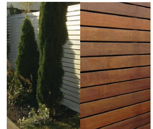
Corner lot / laneway fencing
