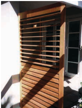
Operable timber louvres for sunshading and privacy
