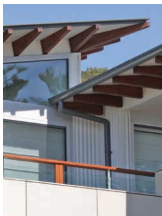
Detailing under eaves and circular downpipes
