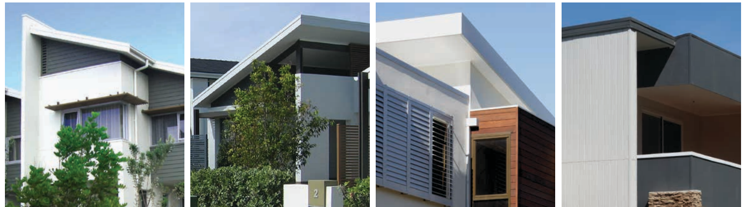
Simple roof forms and lightweight materials
