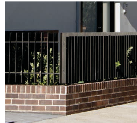
Corner lot fencing - low brick wall with metal blades above
