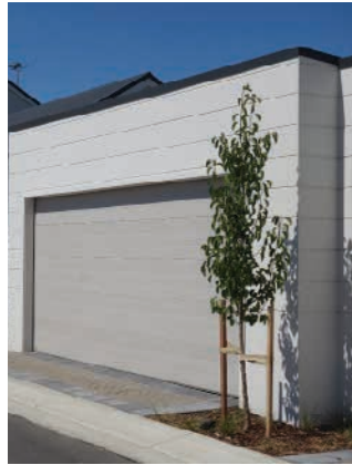
Paving and landscape between garage and laneway
