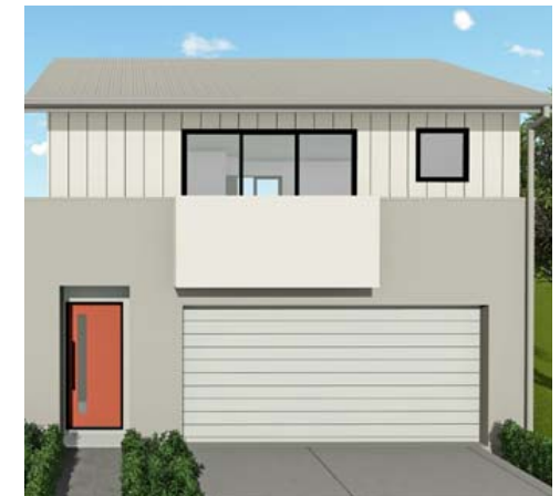
Studios above garages (Fonzie flats)
